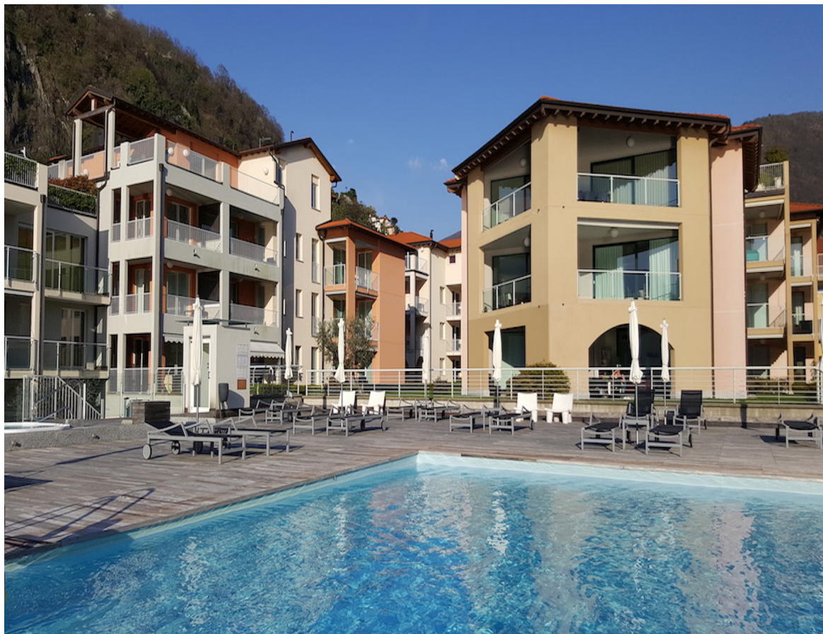
View of apartment exterior
