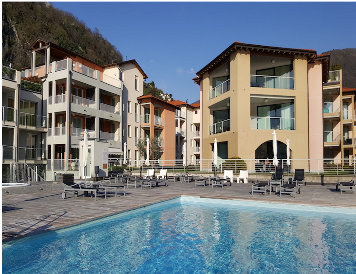
View of apartment exterior
